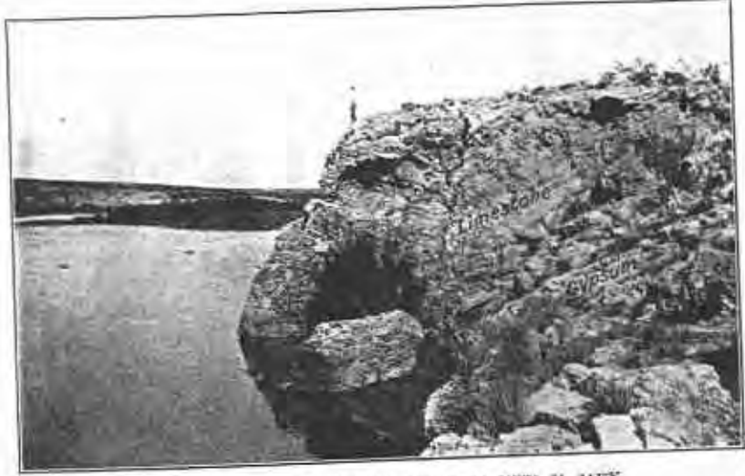
A. PECOS RIVER AT RED BLUFF DAM SITE, N. MEX. Showing dolomitic limestone resting on gypsum. The limestone dips steeply to the east (left) because of slumping due to the removal by solution of some of the gypsum. Photograph by W. T. Lee.
